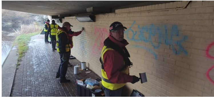
Volunteers removing graffiti in Woking (before)
