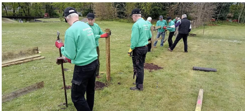
Replacing the fencing around the Mychett camp site
